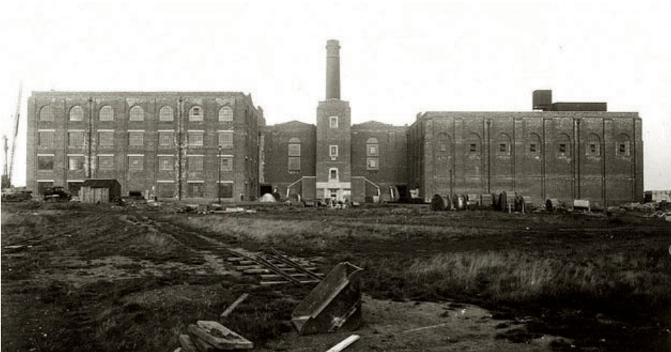
1920s mill buildings at Kemsley Paper Mill. Image provided courtesy of D. S. Smith Kemsley paper Mill.
