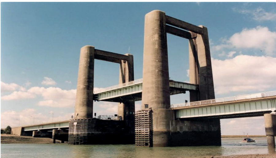
The 1959 Kingsferry bridge with transporter platform raised. (a non-designated heritage asset)
