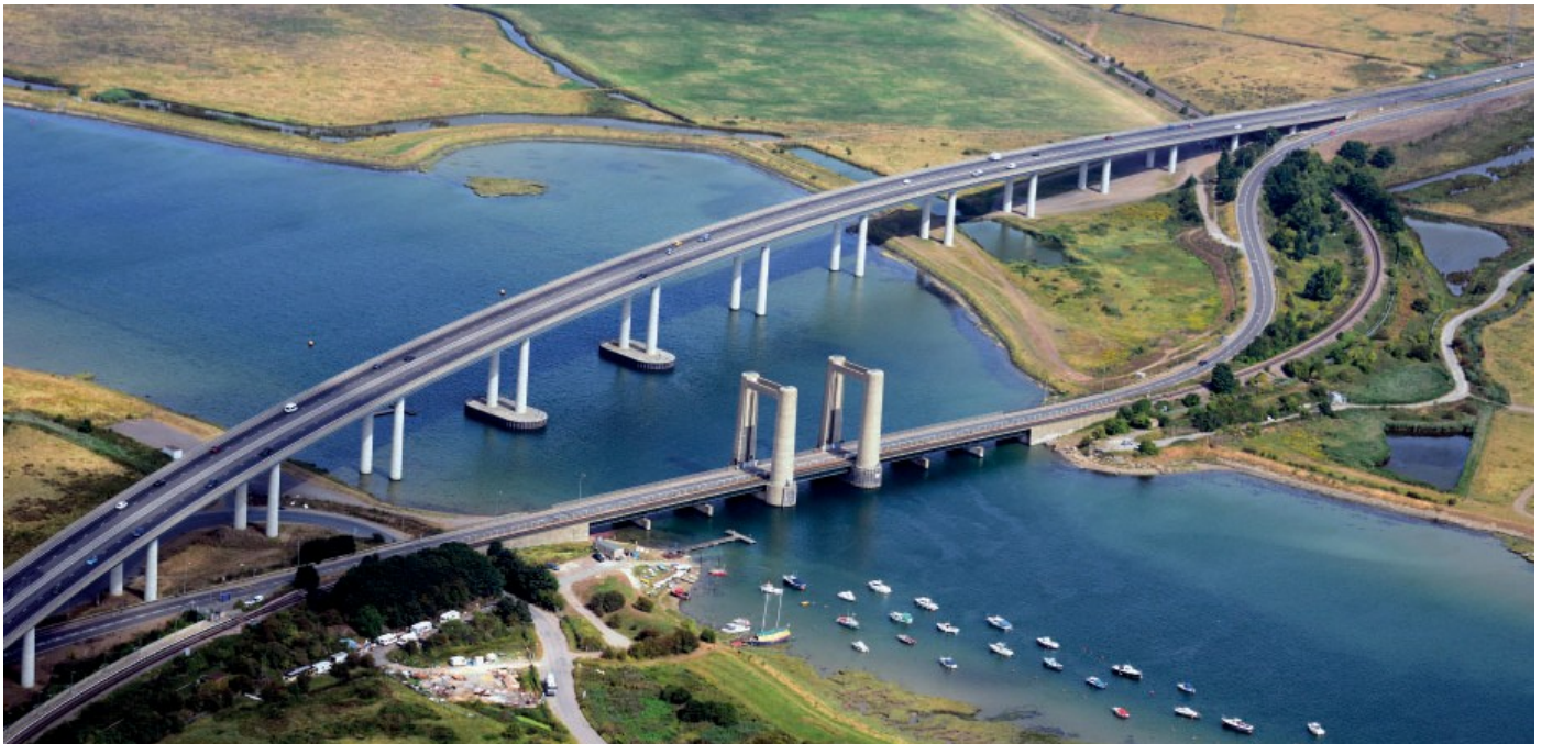
Image of the new Sheppey Crossing, with the Kings Ferry Transporter Bridge in the foreground: two pieces of key 20th and 21st century transport infrastructure linking the island and mainland parts of Swale Borough.
