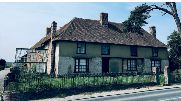
Radfield House, Teynham – at risk grade II listed building
