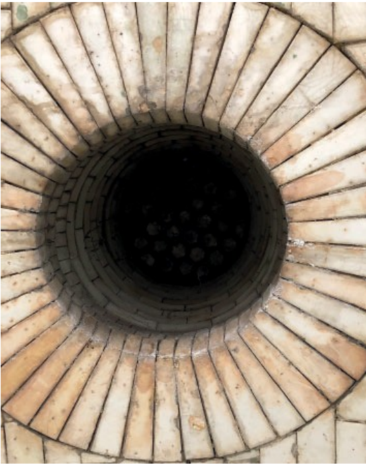
Tiled underpass feature at Faversham Station (a grade II heritage at risk listed building).
