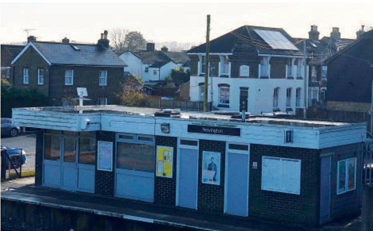
The modern replacement station and adjacent Victorian
